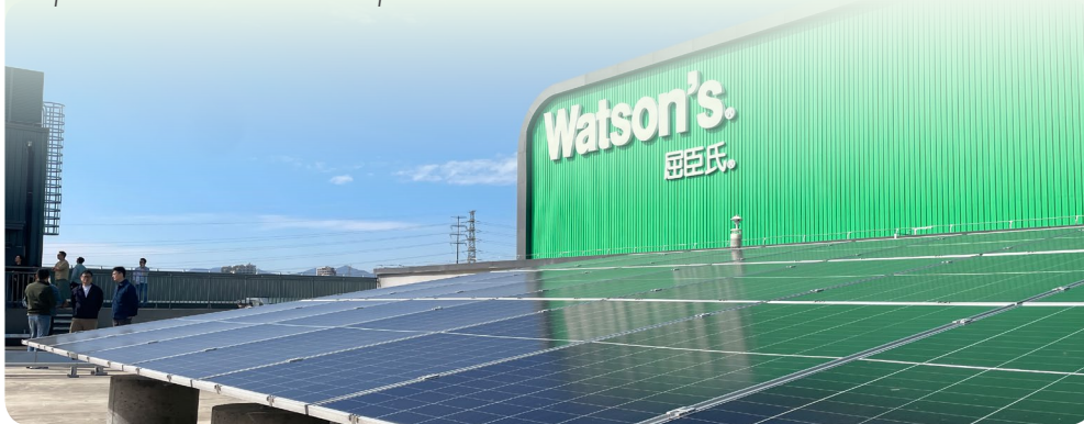
Operations with on-site solar panels installed
